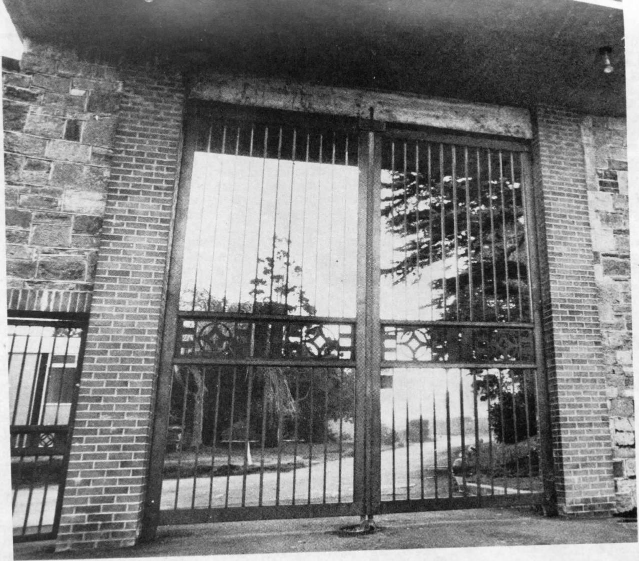
The Central Mental Hospital . . . Martin Dolphin is confined for unspecified 'treatment.'
