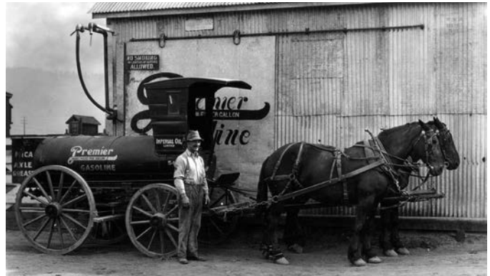
Photo: Kamloops substation with horse-drawn tank wagon, City of Vancouver Search Archives
