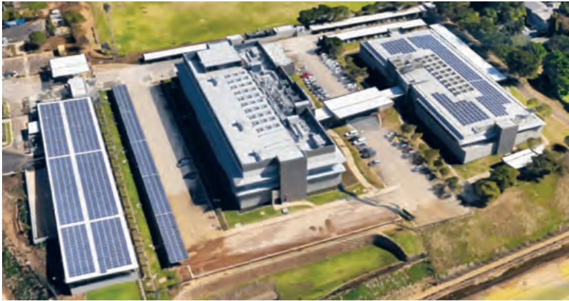
At its office compound in Pretoria, South Africa, USAID has installed solar panels to reduce its energy consumption-related carbon footprint and to increase its climate resilience and energy security, especially as South Africa continues to implement rolling blackouts due to energy shortages. PHOTO: USAID
