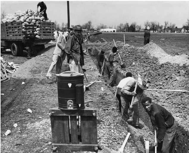
Building site with whites on one side and African Americans on the other. (c. 1950)
