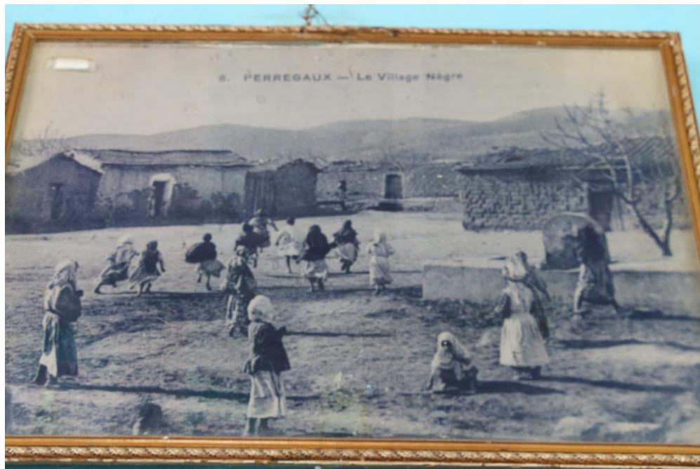
Figure 1: Village Nègre in Perrigaux, photo hanging in zāwīya .
