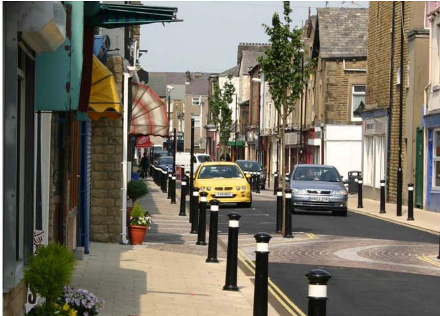
Completed Yorkshire Street public realm works
