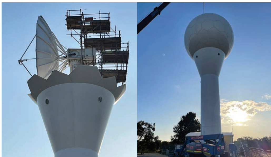
Dome scaffolding at Serpentine (left) and completed Serpentine dome (right).
