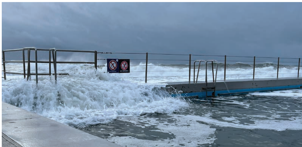
Coastal inundation at The Entrance, New South Wales
