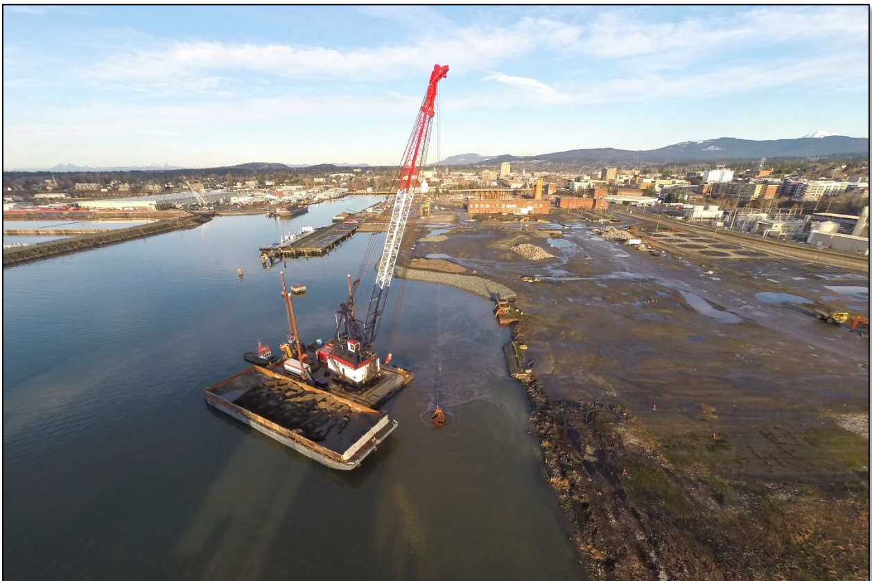
The Whatcom Waterway cleanup project removed 111,450 cubic yards of contaminated sediments from Bellingham's downtown waterfront.
