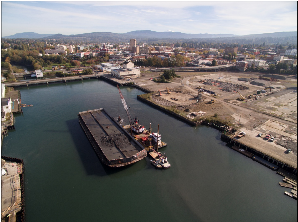
Bulkheads, creosote pilings and concrete debris were removed from the Downtown Waterfront shoreline during the Phase 1 Whatcom Waterway cleanup to support public access and habitat restoration.
