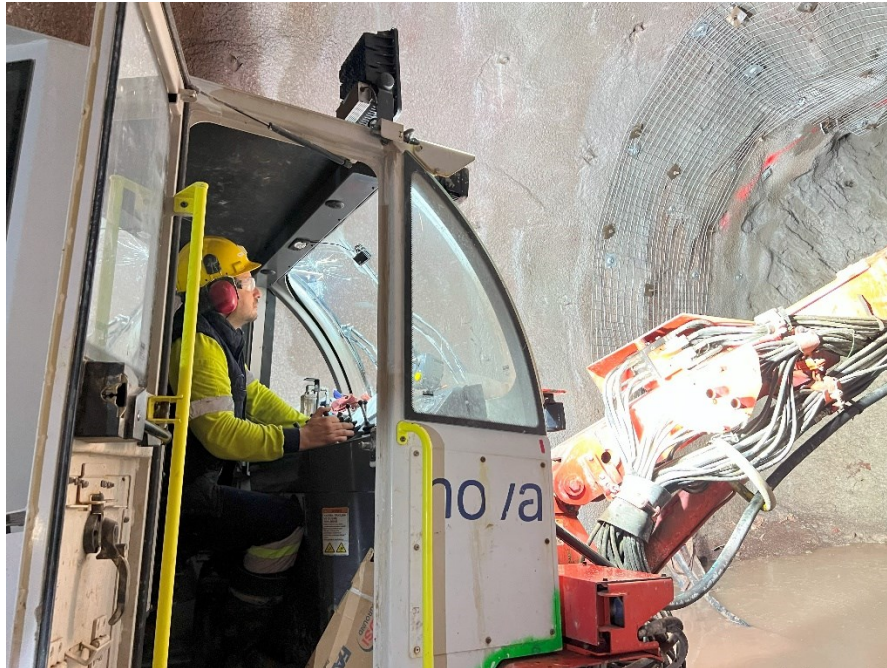
Figure 2: Support installation – bolting, June 2023
