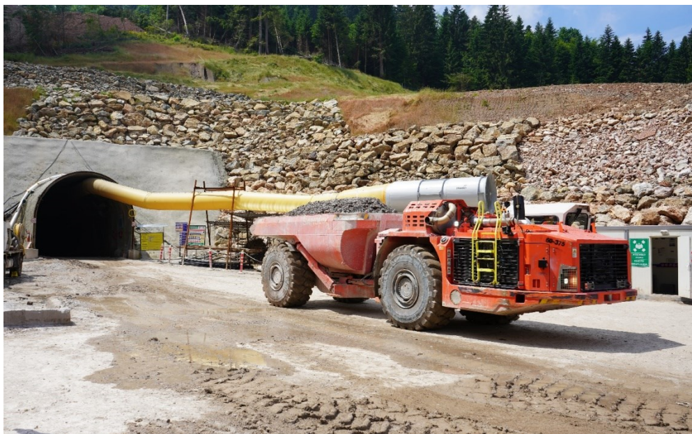
Figure 4: Upper Portal, July 2023
