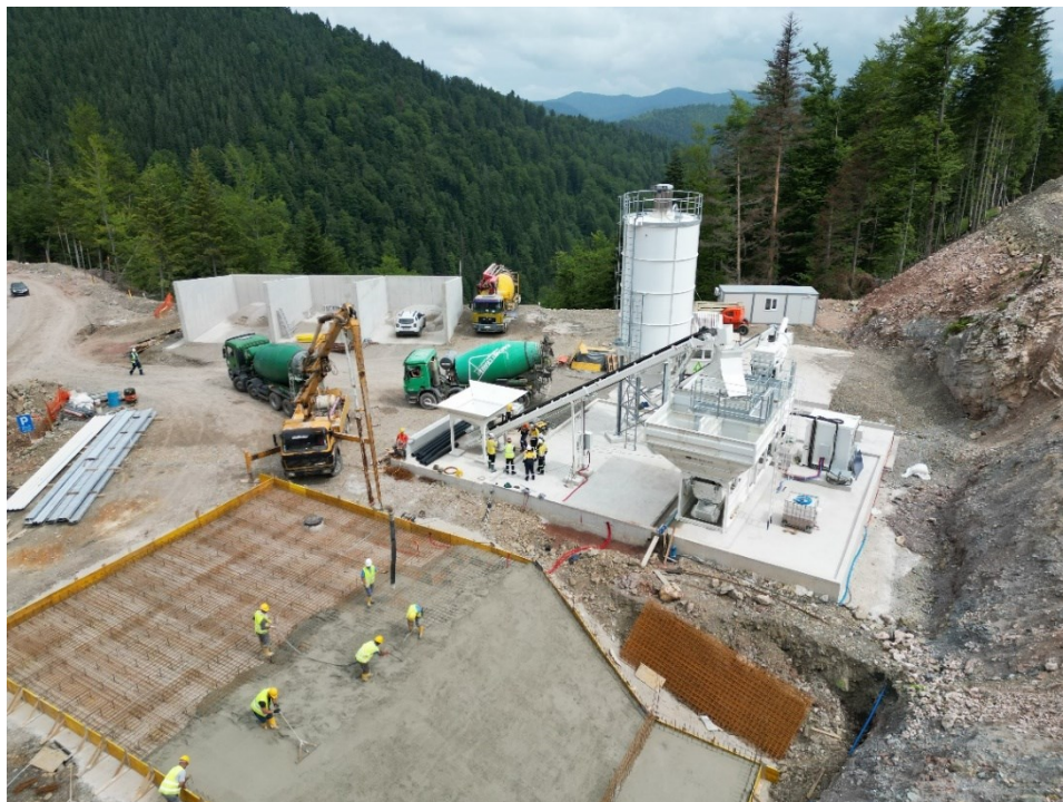
Figure 7: Shotcrete plant Rupice, July 2023
