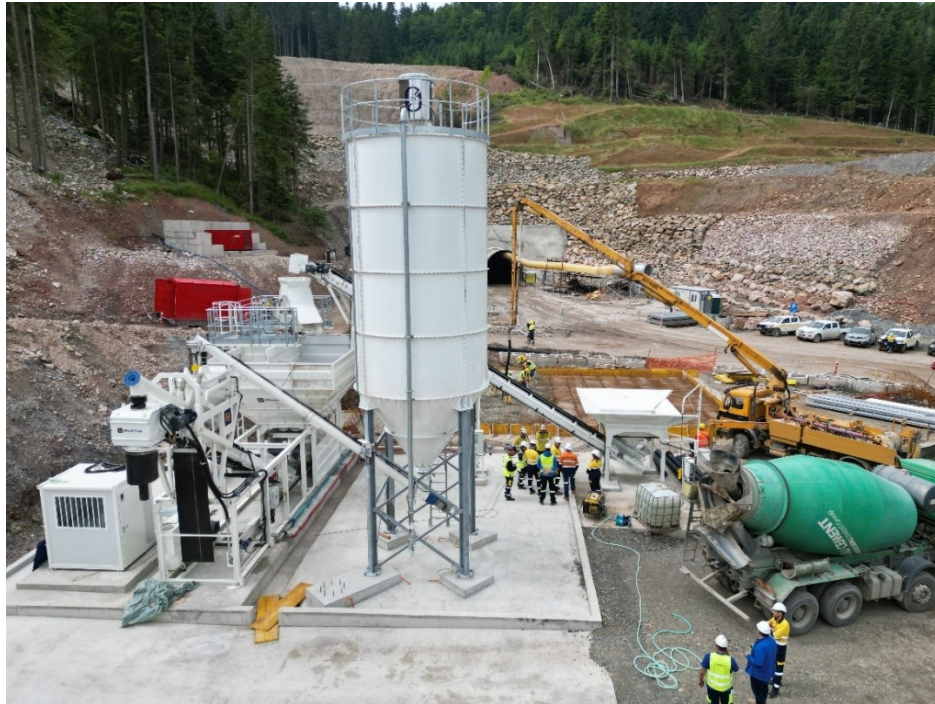
Figure 8: Shotcrete plant Rupice, July 2023
