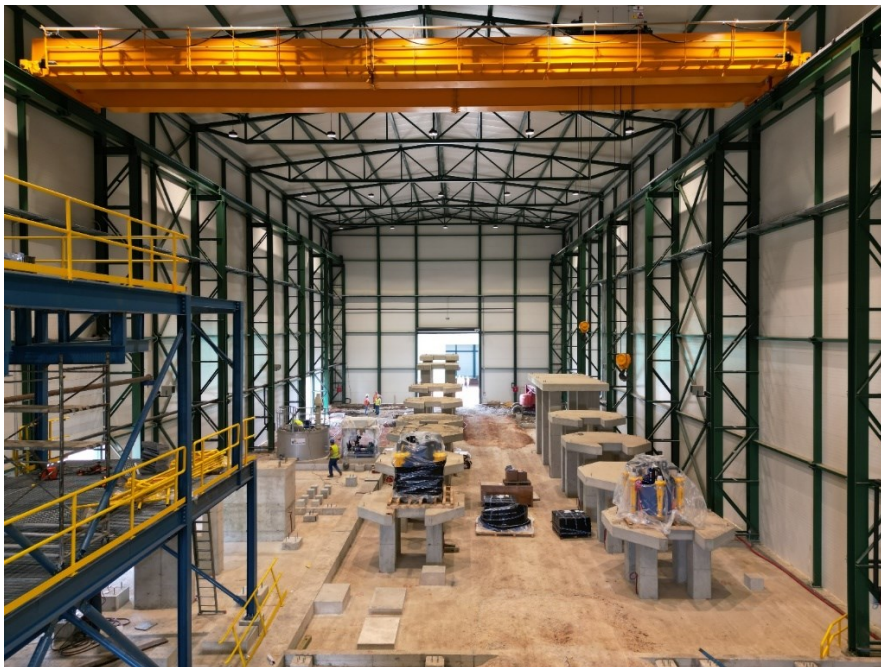
Figure 11: Flotation building, July 2023
