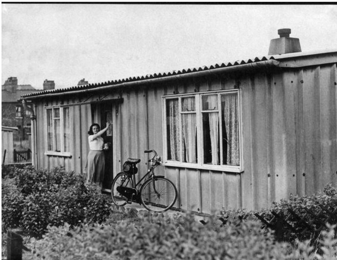
A Phoenix prefab with a simple flat canopy above the front door. Source: Manchester Evening News archive.
