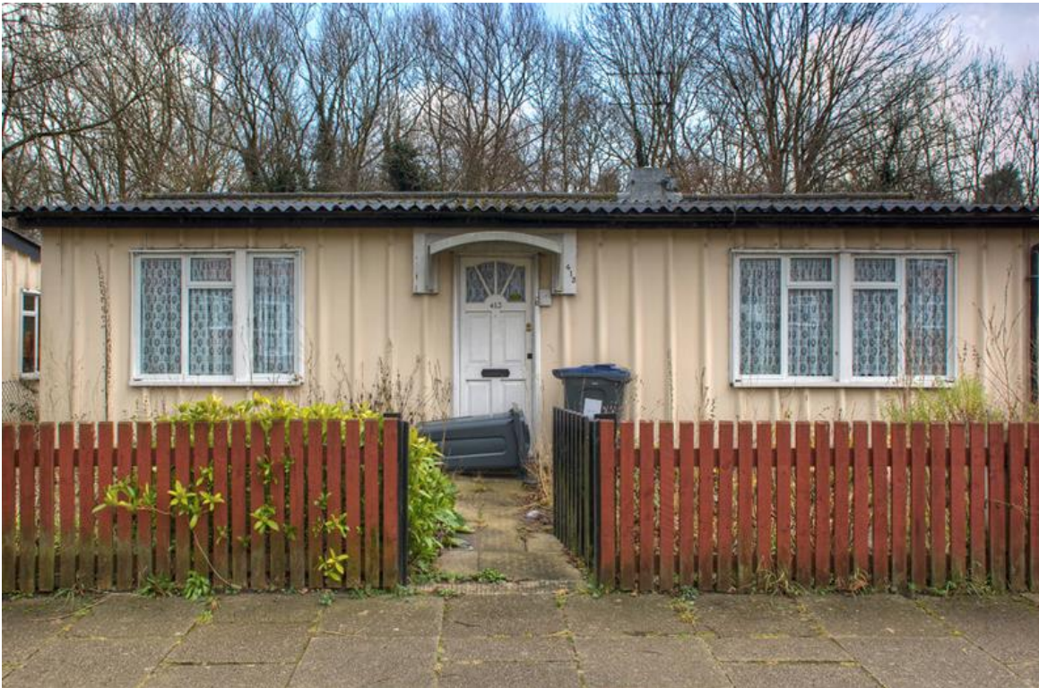
A Phoenix prefab with the characteristic narrow arched canopy above the front door. Source: Gethin Thomas, https://www.flickr.com/photos/speedtree/16167824860/
