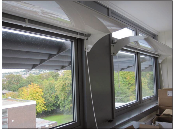
The external brise soleil and internal light shelves.
