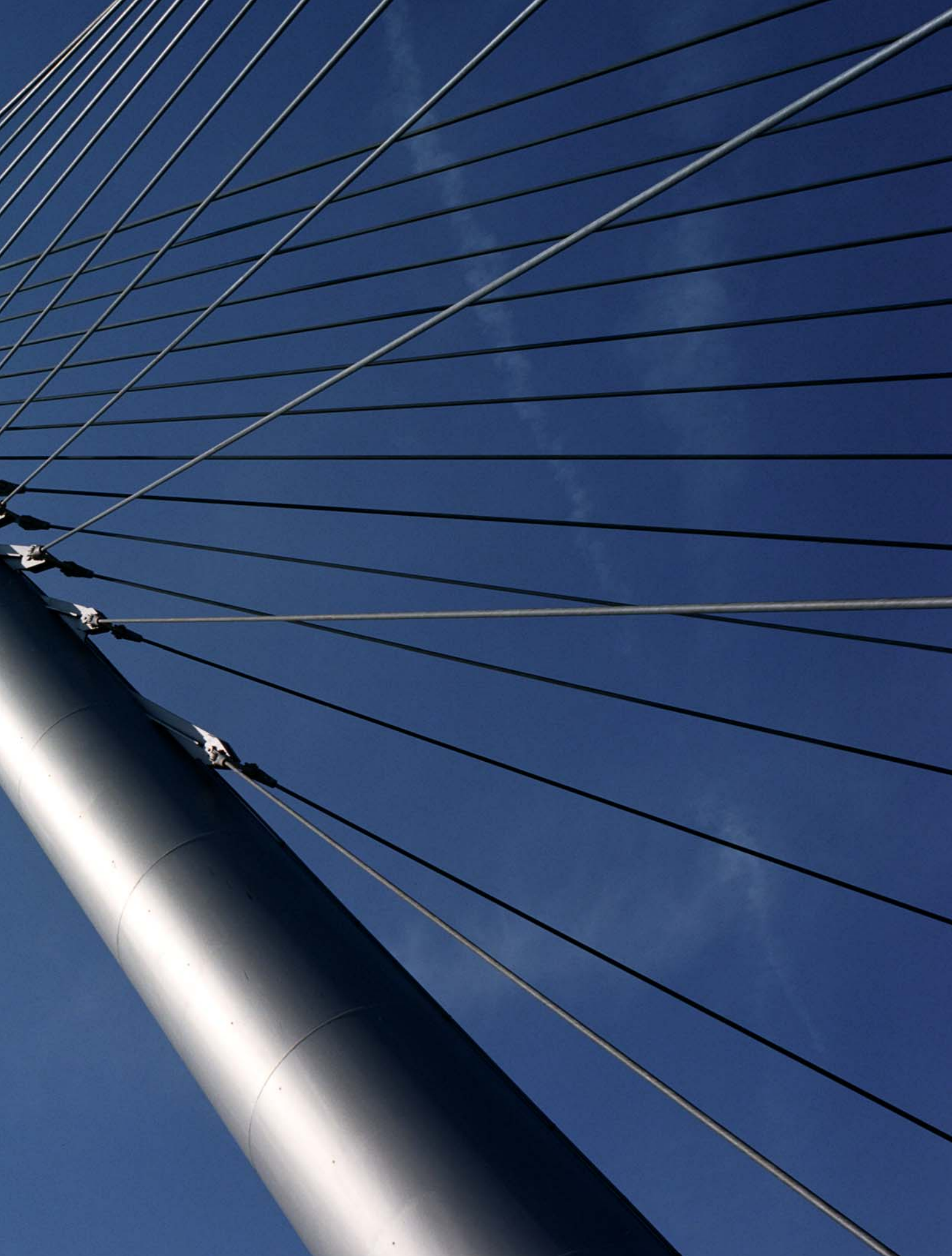
Skyward: the mast above Central Park's yet to be commissioned Metrolink station.
