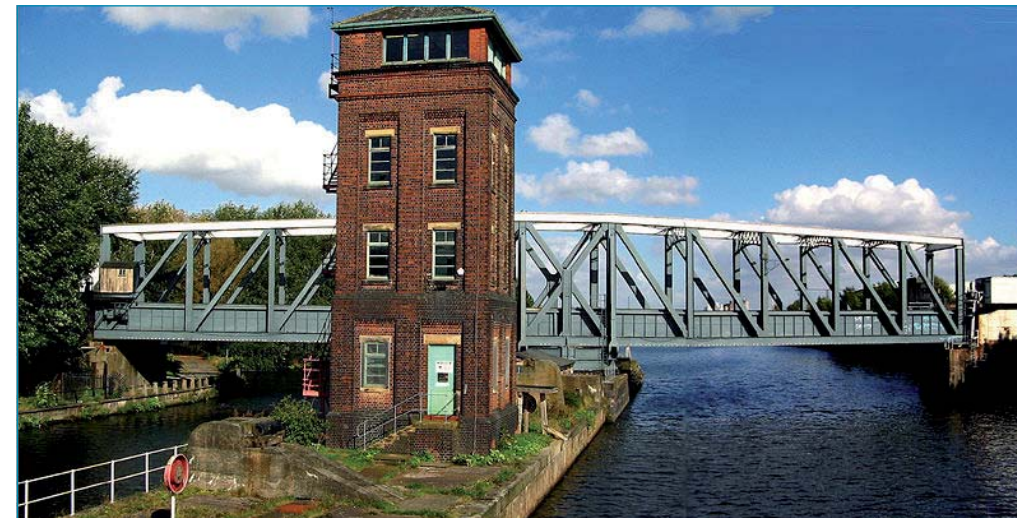
16 The Barton Swing Bridge, Closed to Ships
