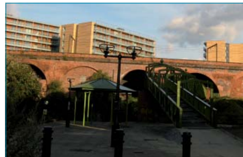
30 Foot Bridge across Canal
