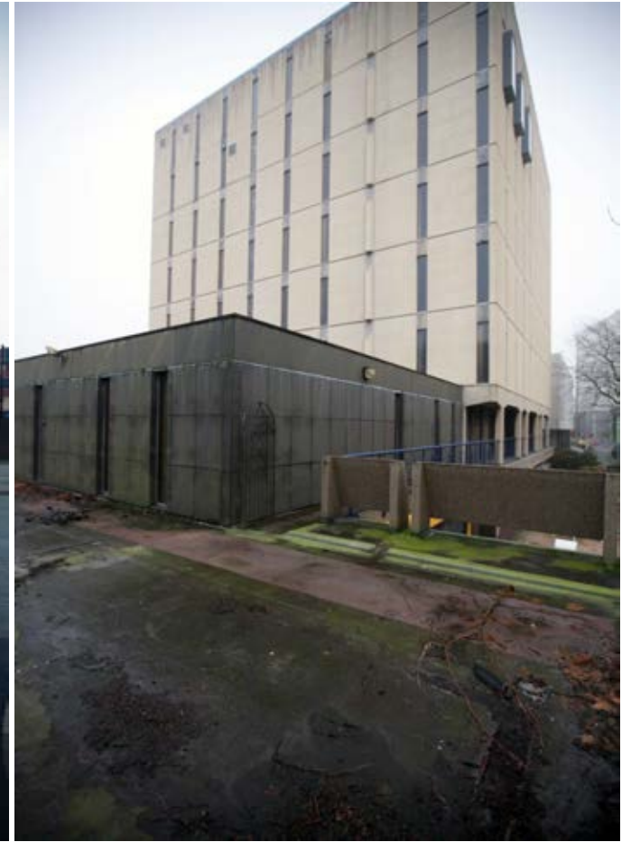
Preston Police Station, 1971.
