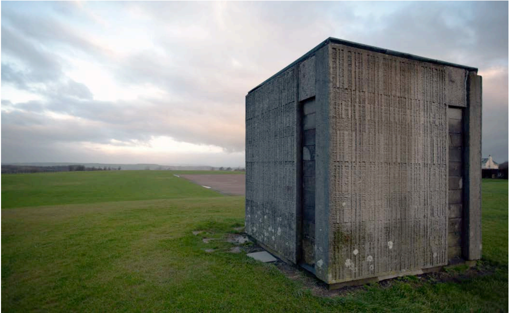
Prototype concrete panel assembly on school playing field, Accrington. Source: Author's photograph, January 2012.
