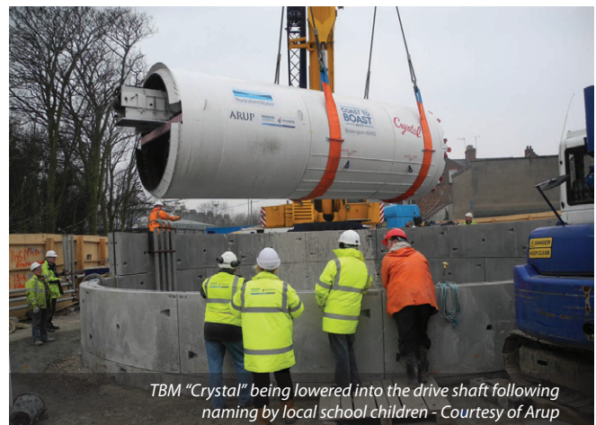
Congested site for Springfield Ave CSO with an existing storm detention tank to the left and a highway bridge on the right - Courtesy of Arup
