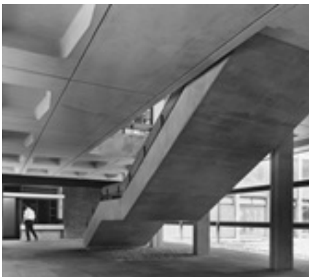
Internal staircase, 1960s
