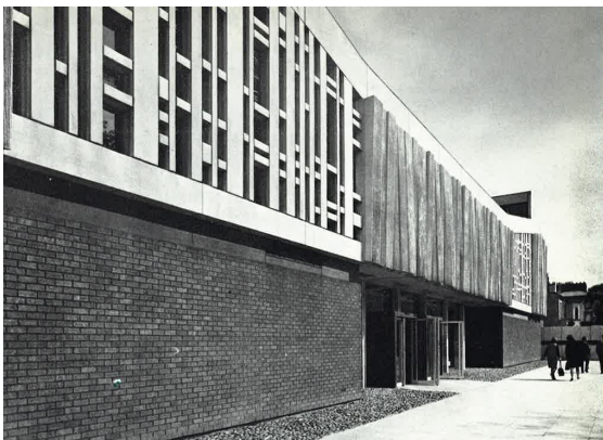
View from Bedford St South, 1964-69
