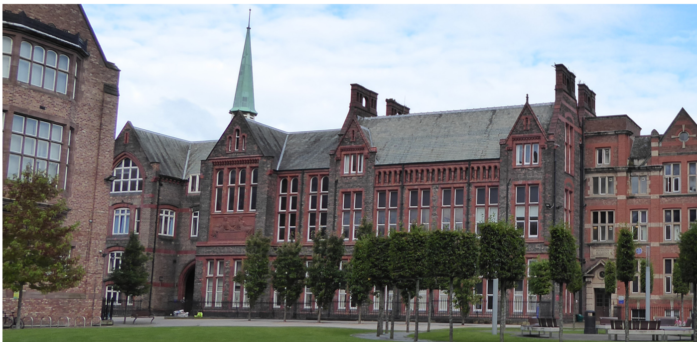
Thompson Yates Building, 2019
