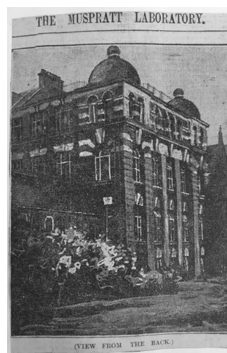
View from Dover Street, date unknown
