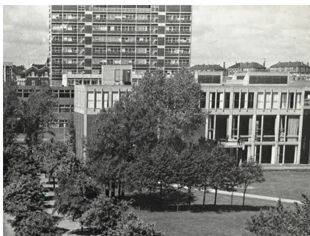
Original rear of building, 1969
