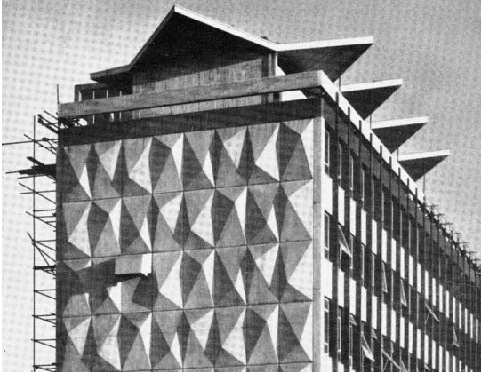
Gable facade and penthouse, 1960
