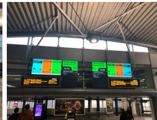
View closer to screens
