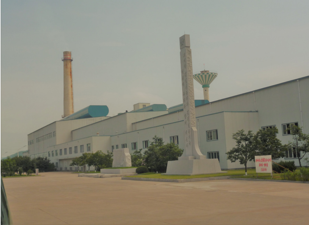
Nampo, North Korea: The Taean Friendship Glass Factory built by the Peoples Republic of China as a socialist solidarity project. Below right: The hi-tech factory's control room. The plant's display room proudly shows a photograph (below left) from when the then Chinese president Hu Jintao together with then North Korea leader, the late Kim Jong-Il, visited the plant in October 2005 shortly after its opening. The PRC must step up economic and military co-operation with its socialistic neighbour and completely ditch the sanctions that the imperialist-dominated UN have imposed on the DPRK. Photos: Trotskyist Platform
