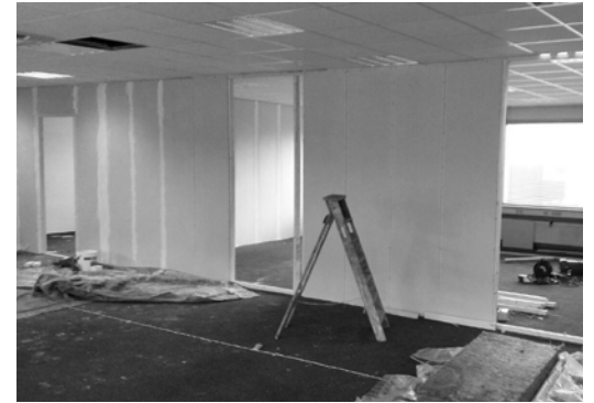
Figure 1: Constructing new walls.
