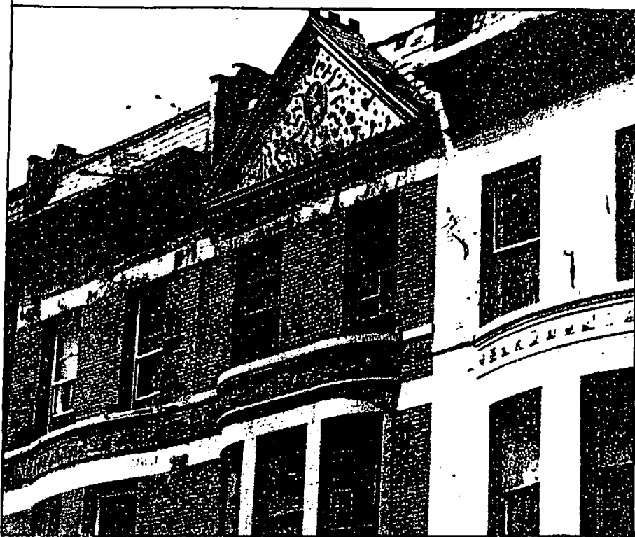
Parcel at 313 W. 136 St. in Harlem. Only the affluent can afford a rehab.
