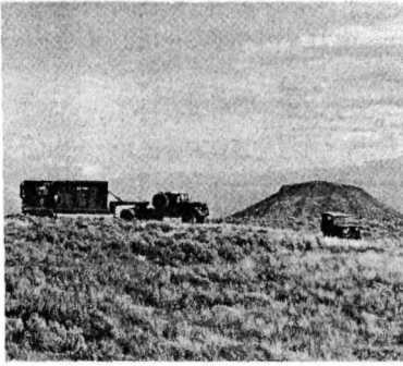
Figure 11 On the right is the ML-1 mobile nuclear power plant in its test configuration. The ML-1 was designed to travel cross-country on a standard military trailer.
