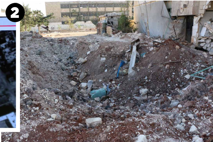
Al Sakhour Hospital, Aleppo, view south, after the October 3 bombing (Source—Yasser Alhaji)
