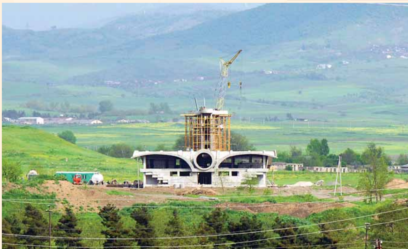
The Stepanakert airport under construction, MKR.
