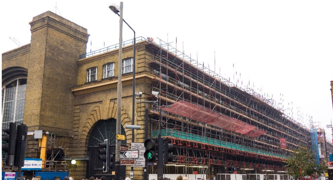
Figure A10.9: Kings Cross Eastern Range Building
