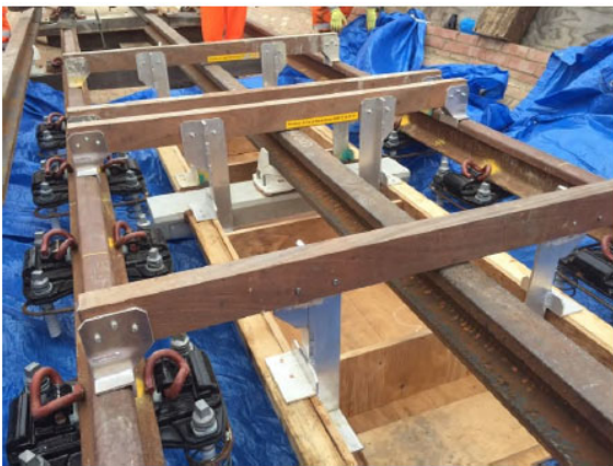
Figure 10-3: Mock-up built to trial method and develop concrete mix and concrete finish for Slipform paved Haunches for HS1 London Tunnels Alliance
