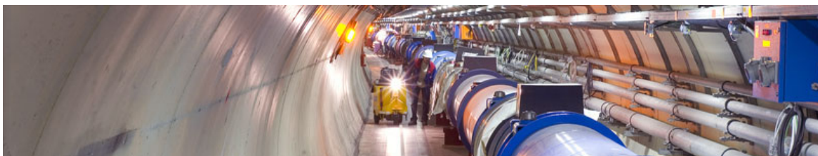
Figure A10.11: CERN Collider Tunnel
