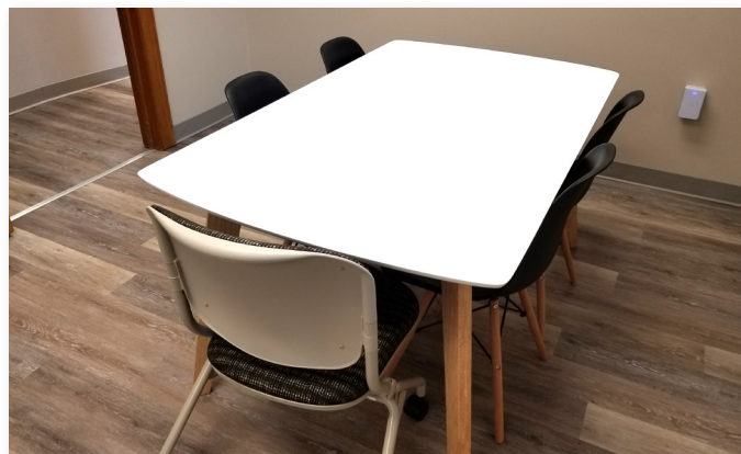
UniFi AC IW AP mounted in wall of common area
