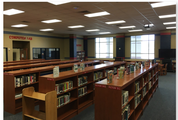
UniFi HD AP installed in high school library
