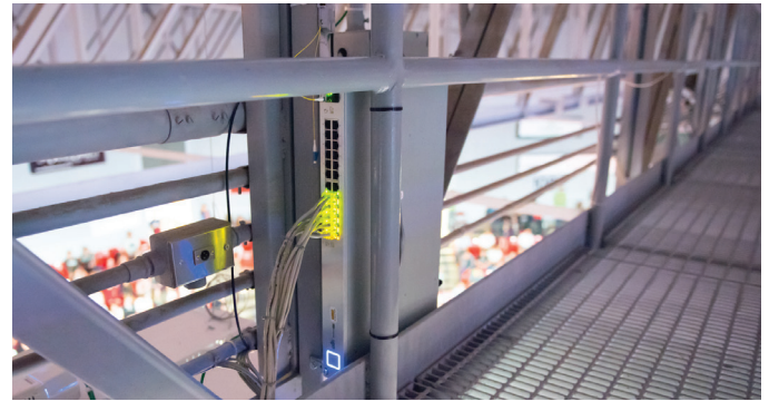
UniFi 16-Port PoE Switch supports multiple APs
