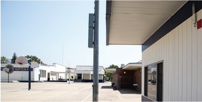
UniFi AP-Outdoor covering basketball courts
