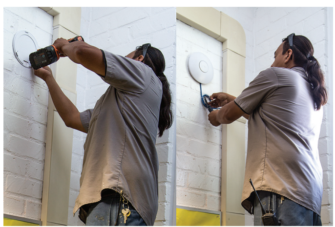
Installing the UniFi AP in a classroom at an elementary school
