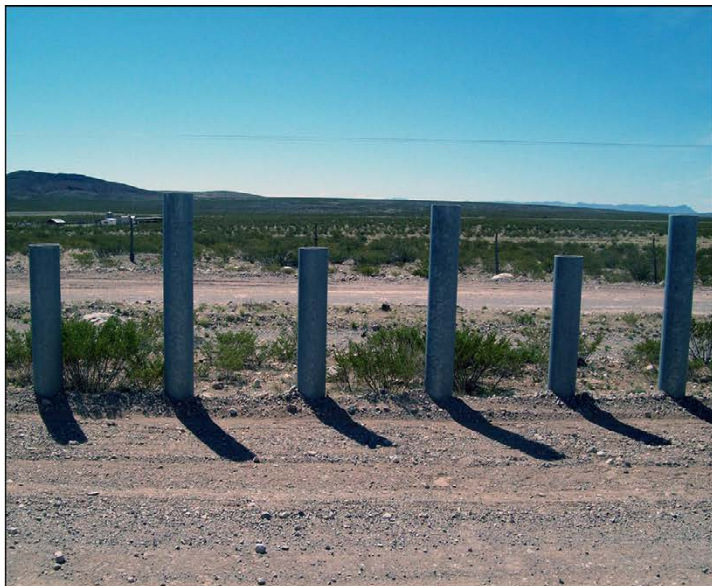
Modern bollard style vehicle fencing
