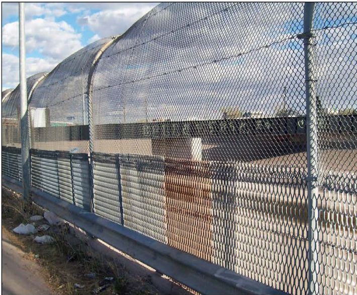
Legacy expanded metal style pedestrian fence
