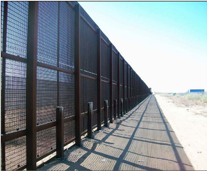
Modern double steel mesh style pedestrian fence
