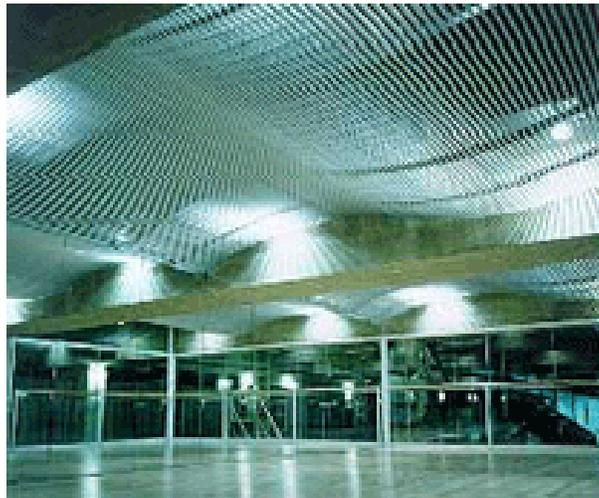
Figure 32. Chilled ceiling panels in Cannons, Covent Garden. Source SAS International
