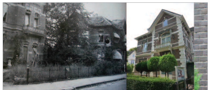
Left: Stationsweg 6 and 8 after the battle. Centre: Stationsweg 8 today. Right: signs of battle damage in the brickwork of Stationsweg 8
