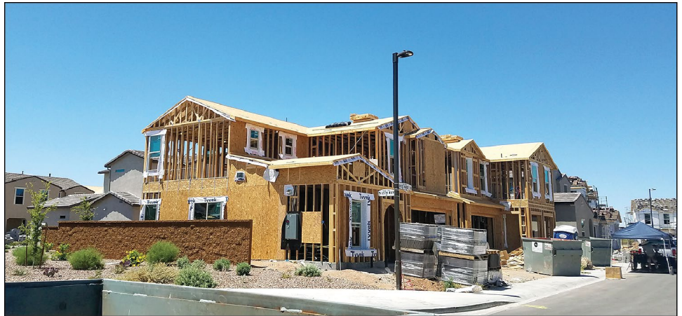
Figure 12: Housing Units Being Constructed by Company that Subcontracts with an H-2B Employer in Maricopa County, Arizona
