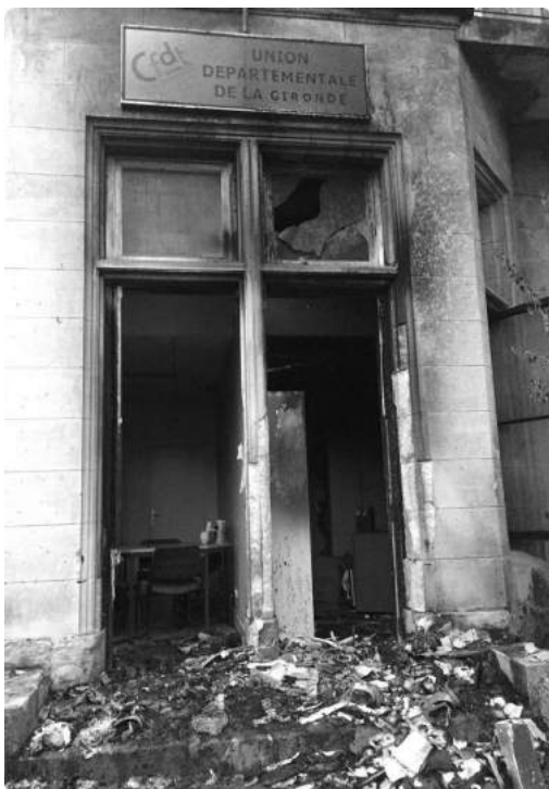
Bordeaux, France: CFTD office heavily fire-damaged a week after the events in Paris
