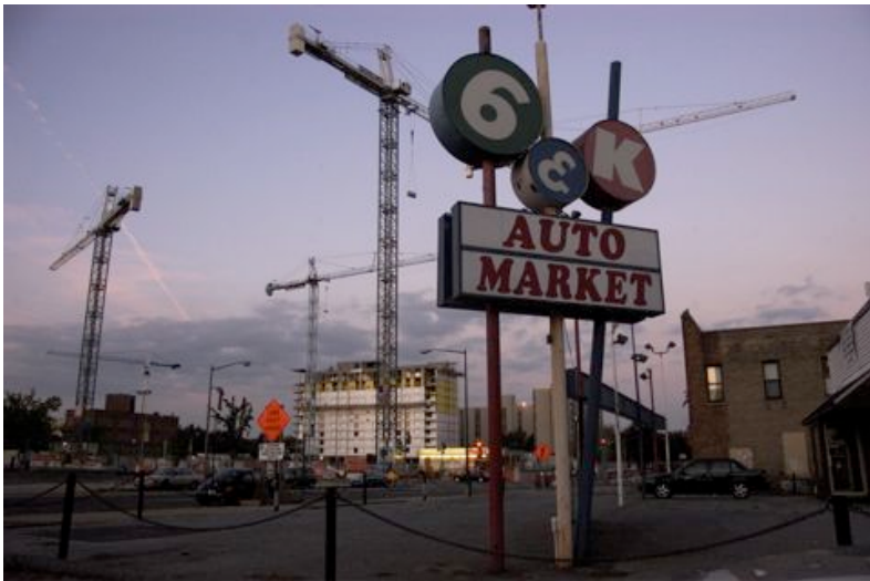
Figure 7: Construction on K Street, NW. Photo taken September 17 2006 by PJ Starr.
