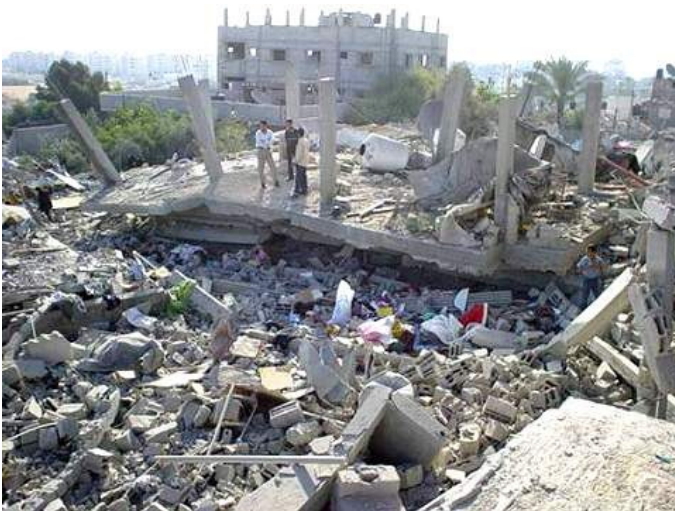
Gaza ruins. The reconstruction of Gaza requires a huge amount of cement and other building material, none of which has been allowed in.
