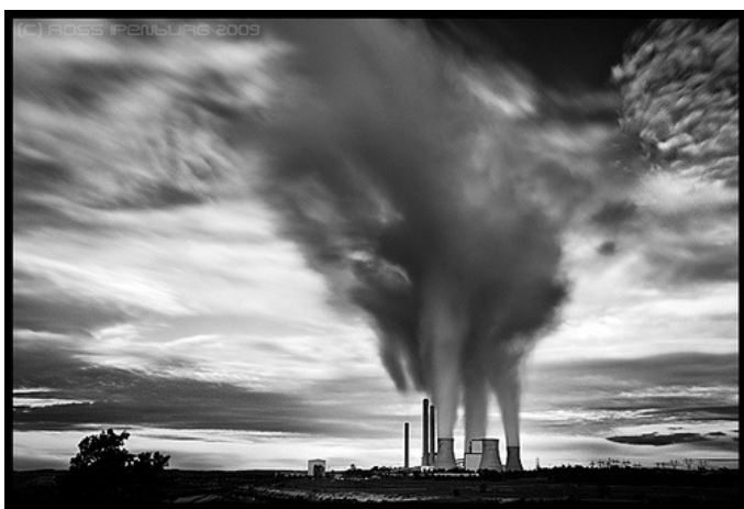
Loy Yang power station. It is not the visible steam but the invisible carbon dioxide that we need to cut
