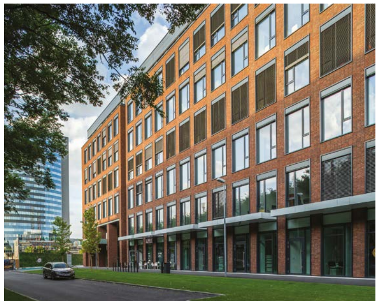
Completed Twin City
