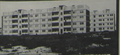
Housing Commission Hall - centre pages
