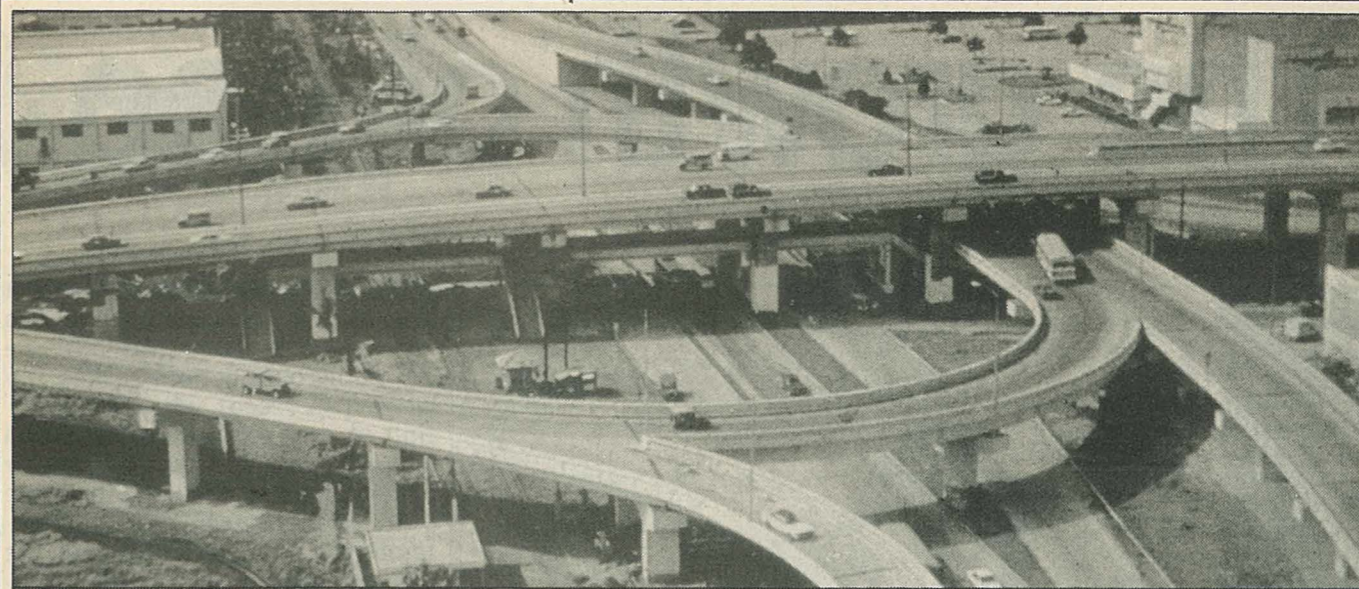
Development in the Philippines — the infrastructures of capitalism.
