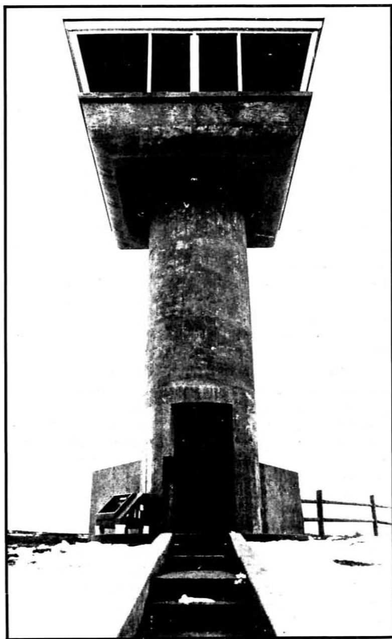
Photo: The Southern Illinoian
