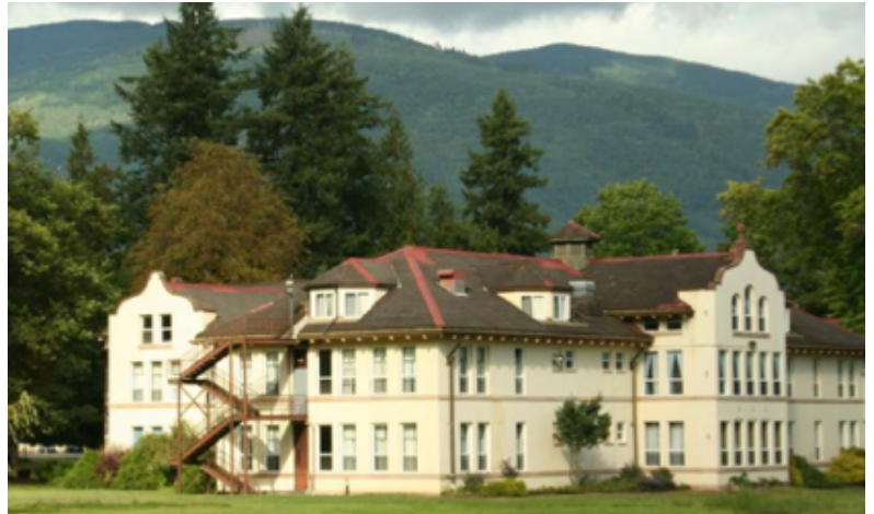
Former Northern State Hospital, 2012.
