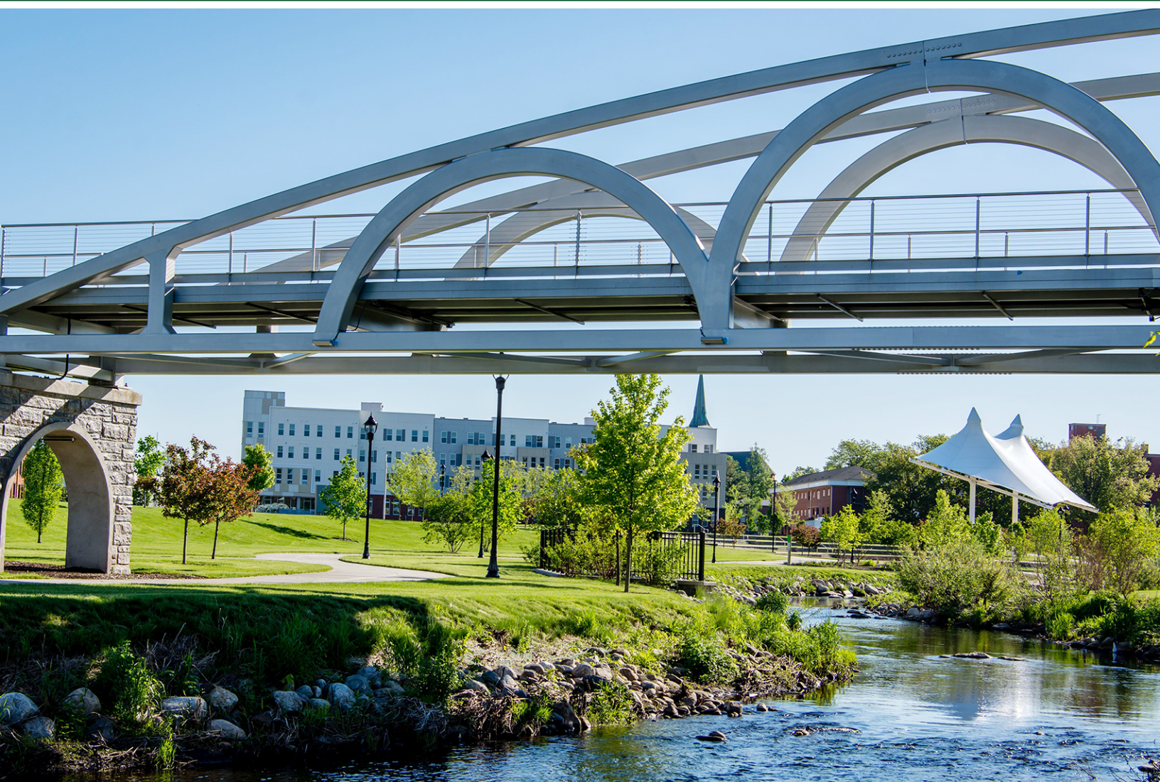
Pedestrian bridge over Harbor Brook at Meriden's downtown Hub site in Meriden, Connecticut. Photo courtesy of Dave Cooley, Making Meriden Business Center.
