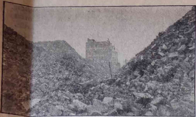
Large areas of London are already reduced to piles of debris and rubble such as the above. This FREEDOM photograph was taken in Aldersgate, in the City.
