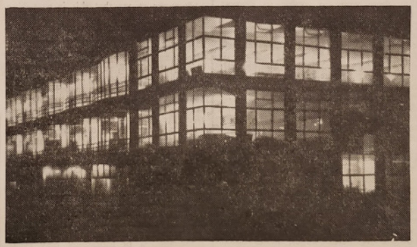
Peckham Health Centre photographed at night, 1947
