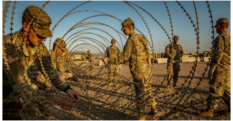
Army's 104th Engineer Construction Co., based at Fort Hood, setting up razor wire near Nogales, Arizona. Photo: Meridith Kohut, TIME November 15, 2018
