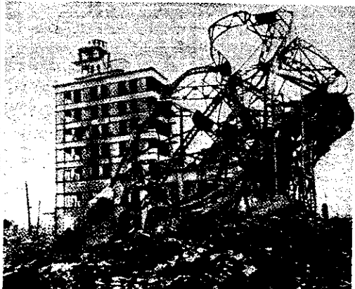
THE SEVEN-STORY steel-framework building in the background of this picture was completely gutted although it was one mile from the centre of the Hiroshima atom bomb explosion. The tangled mass of steel in the foreground was a smaller, lighter-framed building. Help to ban the atom bomb by signing the Stockholm Peace Appeal. (Turn to Page 3 for story on horrors of Hiroshima and Bikini.)
