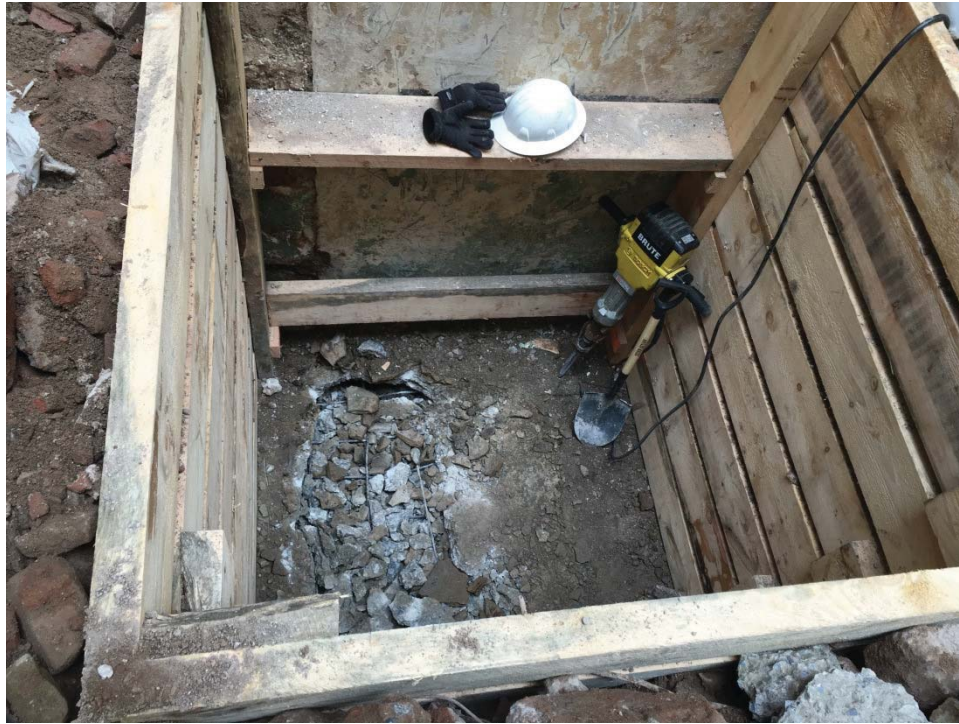
Photo 004: General view of the test pit showing rebar found underneath the 9-inch-thick concrete slab, facing southwest.
