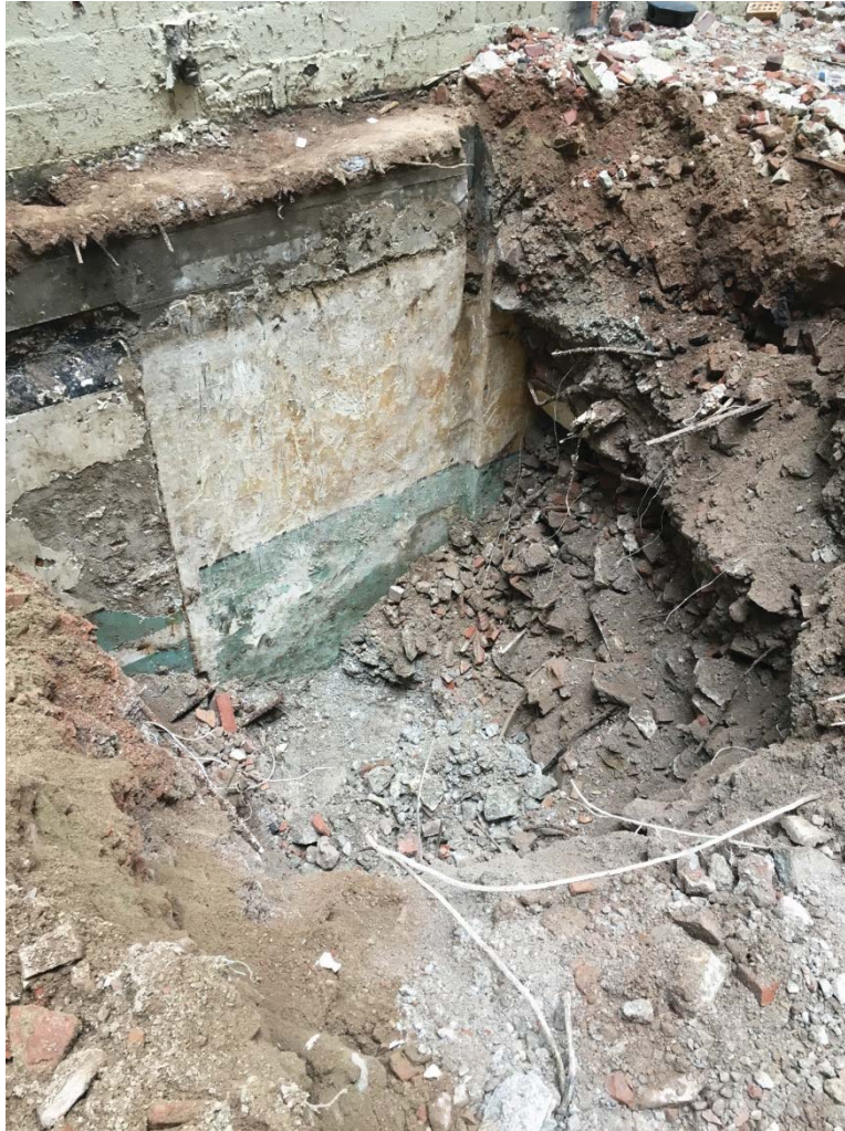
Photo 001: General view of the existing foundation wall, facing southwest.
