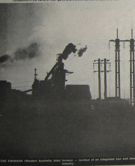
THE KWANANA (Western Australia) blast furnace — nucleus of an integrated iron and steel industry.
