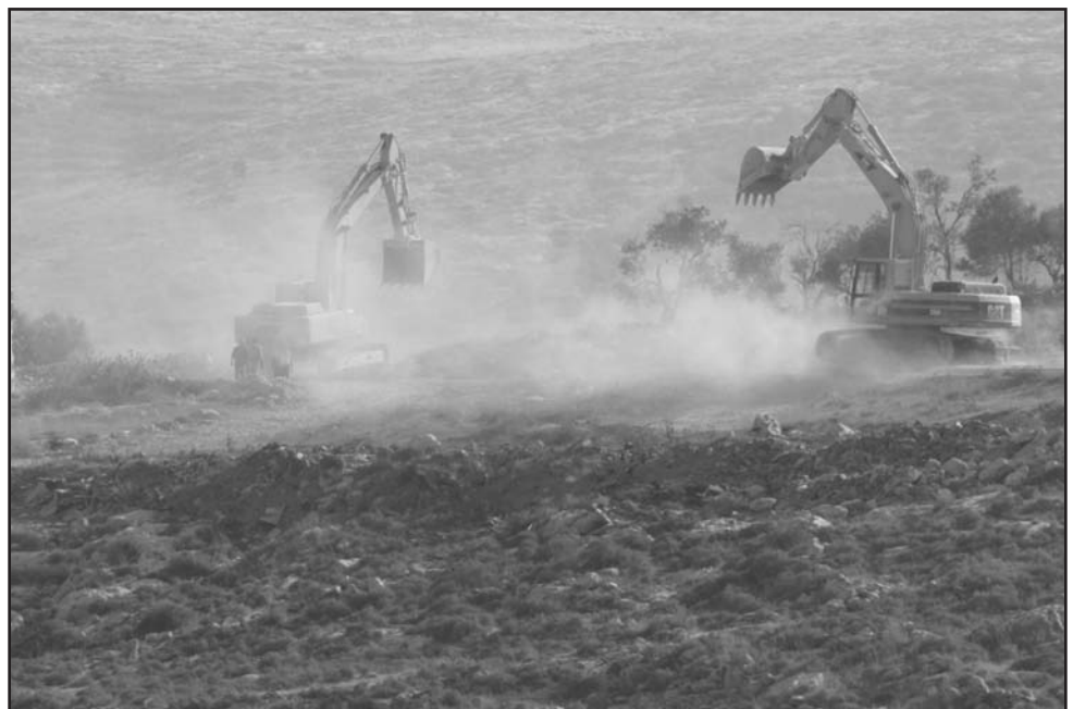
West Bank Wall construction near Bil'in. photo: Jon Elmer
