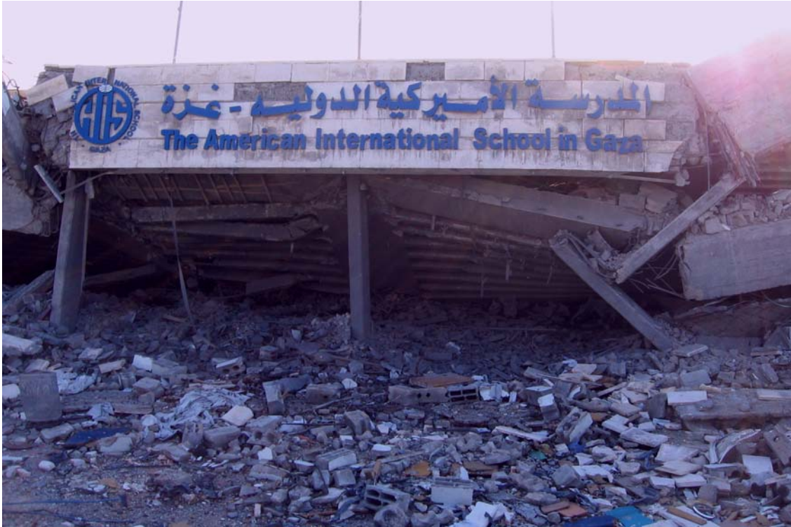
Picture 9: The destroyed American School showing the main building from the street.
