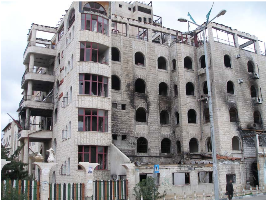
Picture 7: Damage to the Al-Quds Hospital.
