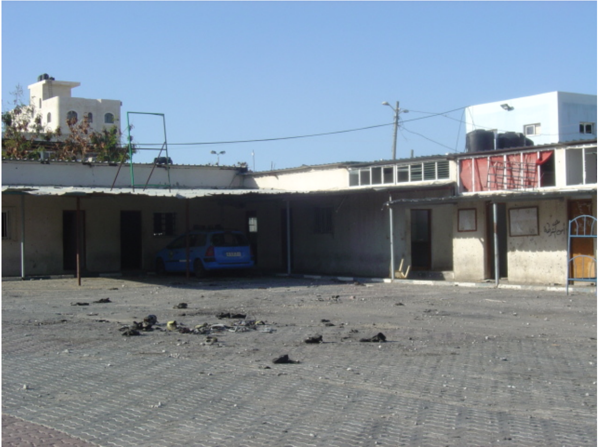
Picture 18: The parade yard where the first shell landed. Remnants of clothing and shrapnel were still present on the site when the Committee took this picture.
