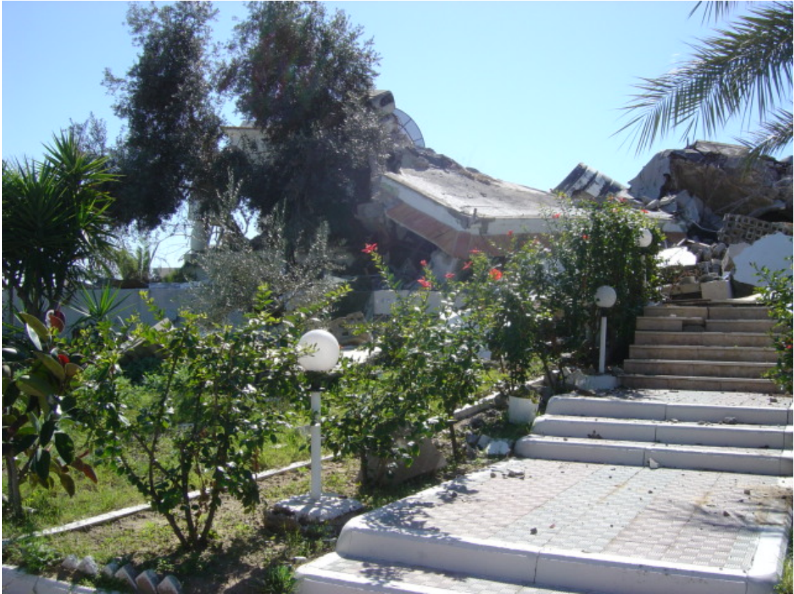
Picture 16: The destroyed President's Guest House.
