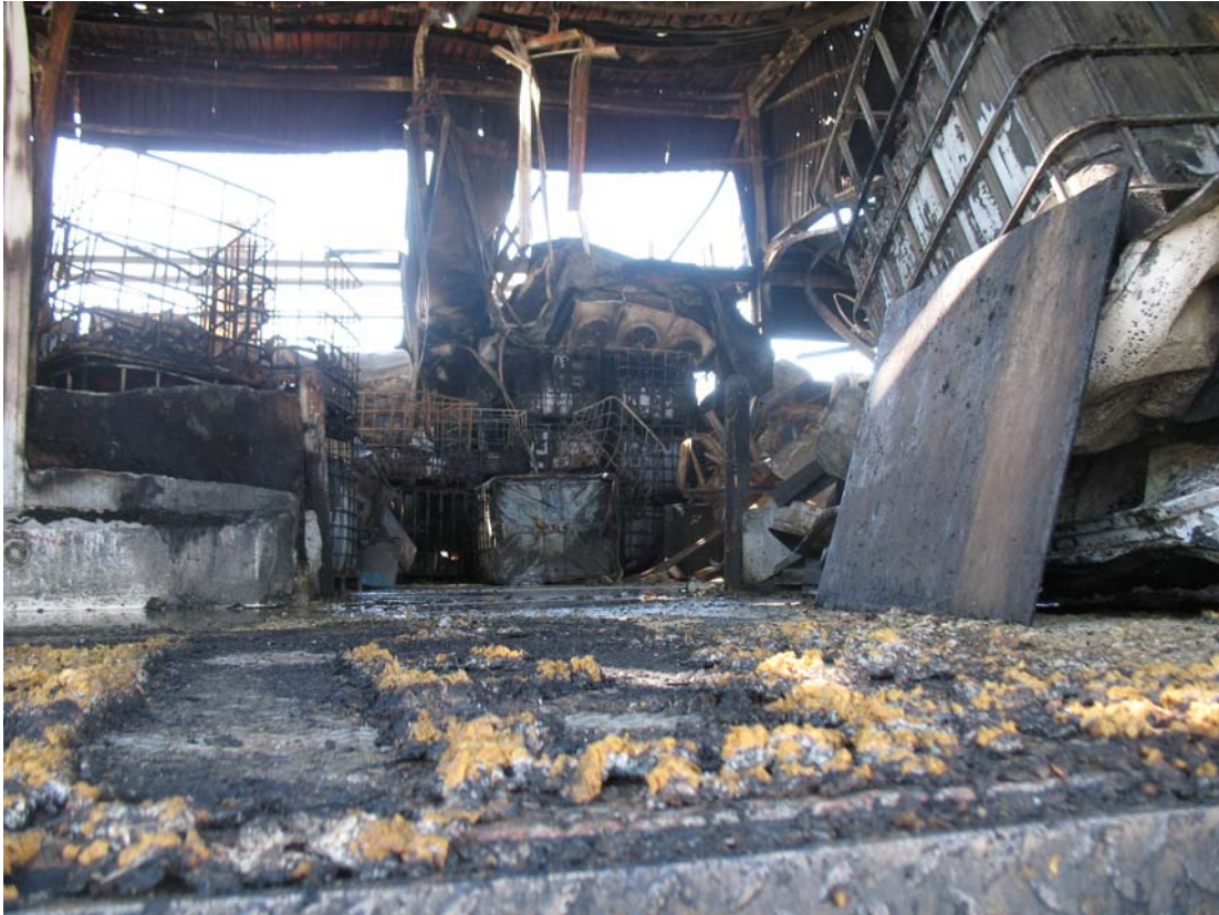
Picture 22: One of the destroyed buildings at the juice factory.
