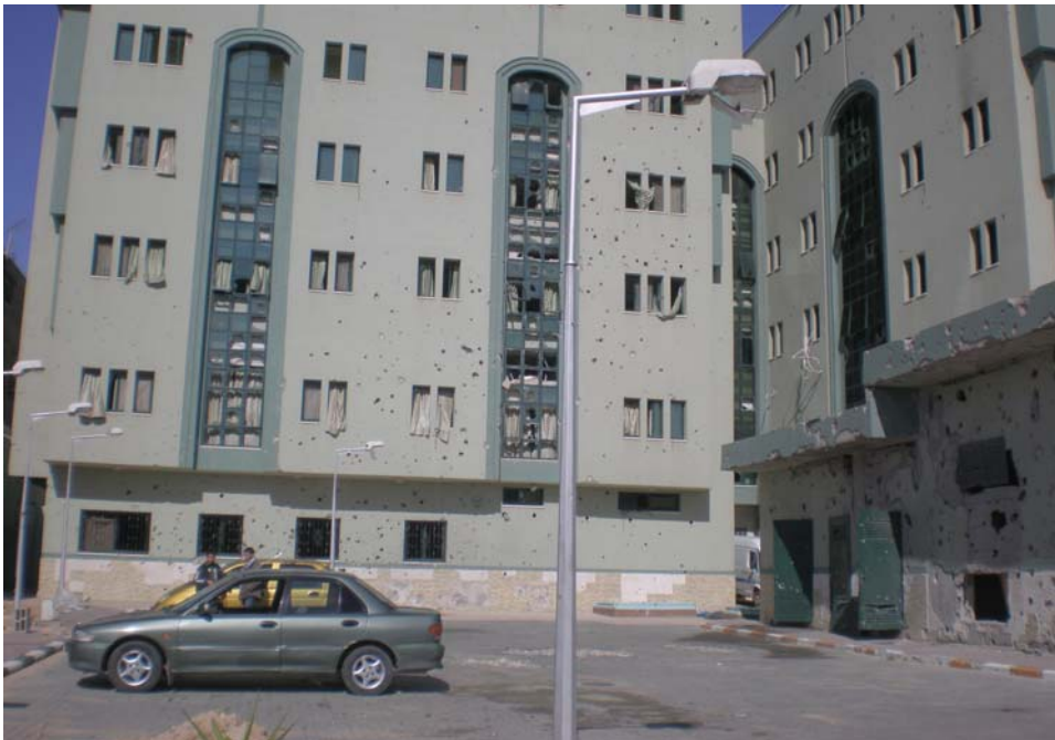
Picture 6: Damage to the new buildings of the Al-Wafa Hospital.
