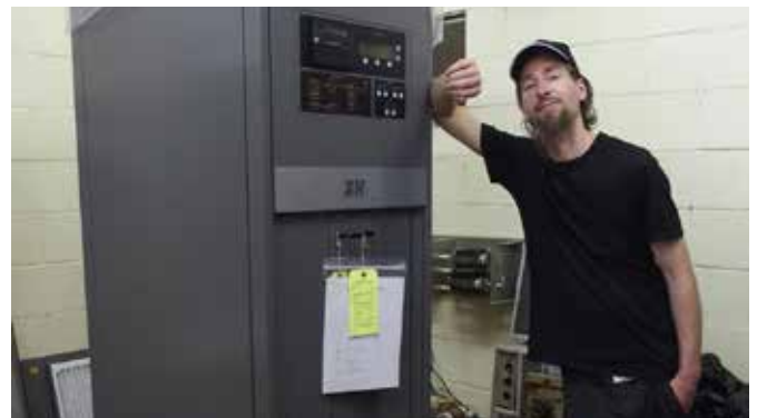
3CR technician Riah Williams installing our new transmitter
